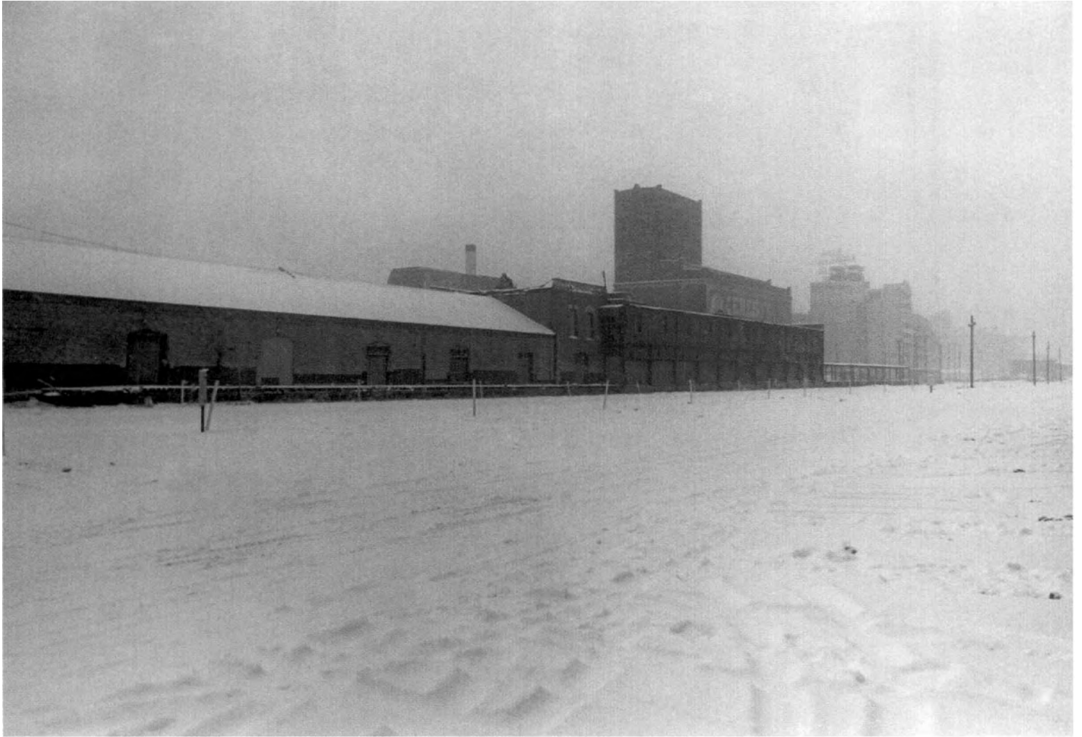
MILWAUKEE ROAD FREIGHT HOUSE AND CERESOTA ELEVATOR, WEST SIDE MILLING DISTRICT, MINNEAPOLIS, 1988
